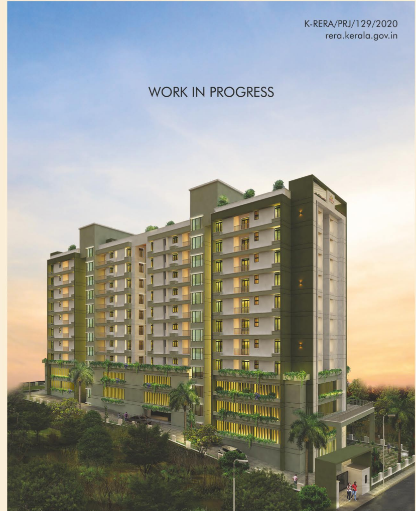
QUEENS COURTYARD Off Medical College, Calicut
